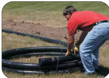
2 Decoil to the next fixing band. Continue this procedure until decoiled.
