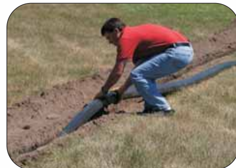
3 Place ThermoPEX into trench.
