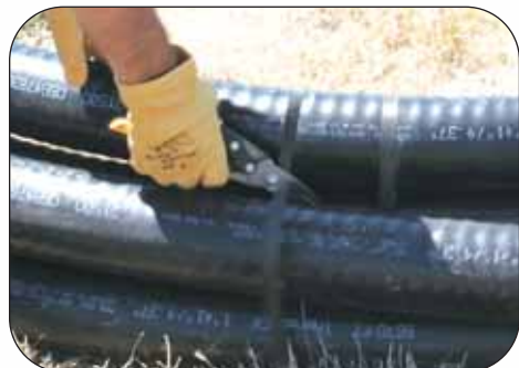
1 Cut the three outermost fixing bands.
