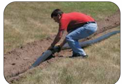
3 Place ThermoPEX into trench.
