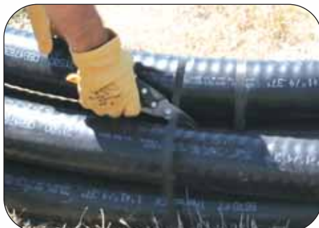
1 Cut the three outermost fixing bands.
